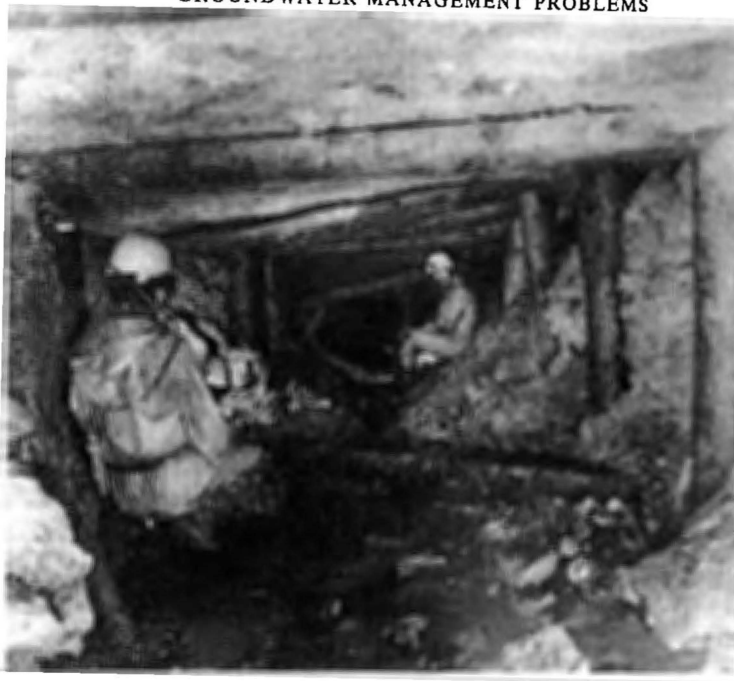
FIG. 7. Free drainage in mine workings abandoned in 1956. Closure of the adjacent mined galleries by swelling of the seat earth has occurred, and the stone retaining walls on both sides of the roadway have collapsed. Seat earth is being eroded by the small stream keeping the roadway open, below the intact Pennant Sandstone roof.
